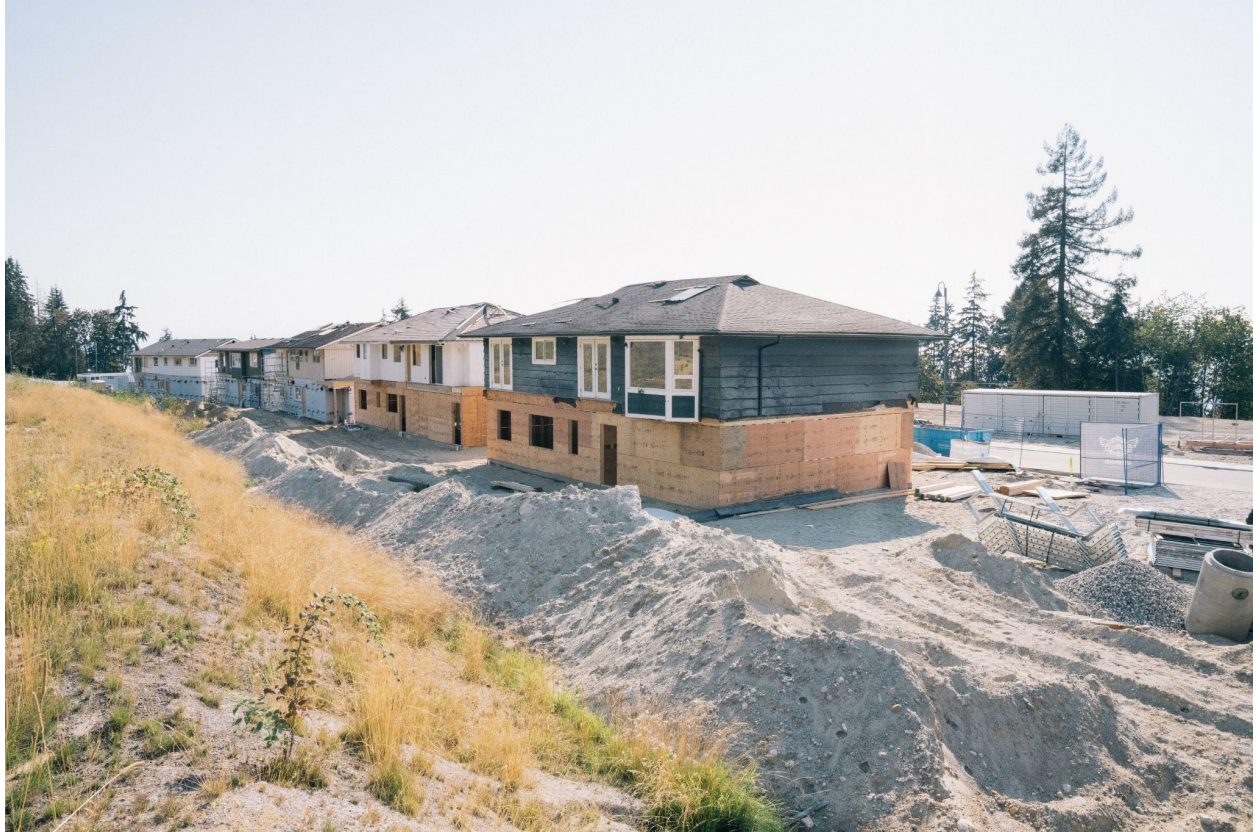
Basement suites added to relocated homes.
