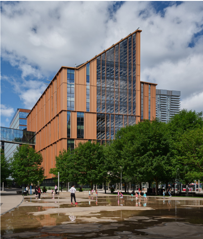
EXTERIOR VIEW OF LIMBERLOST PLACE FROM SHERBOURNE COMMON PARK
