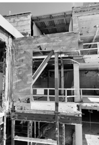
New openings framed in extending construction
