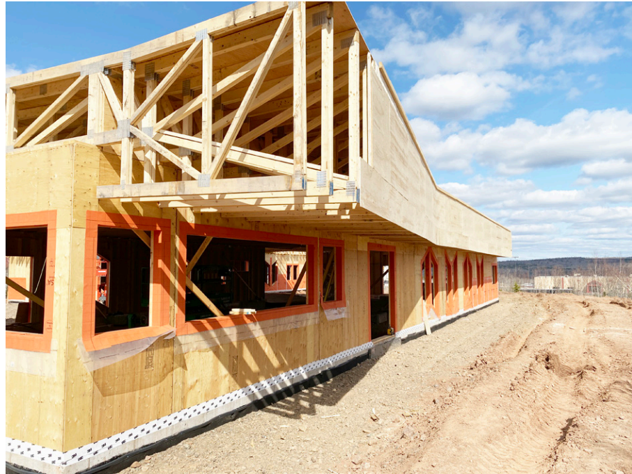
Regionally harvested wood frame structure.
