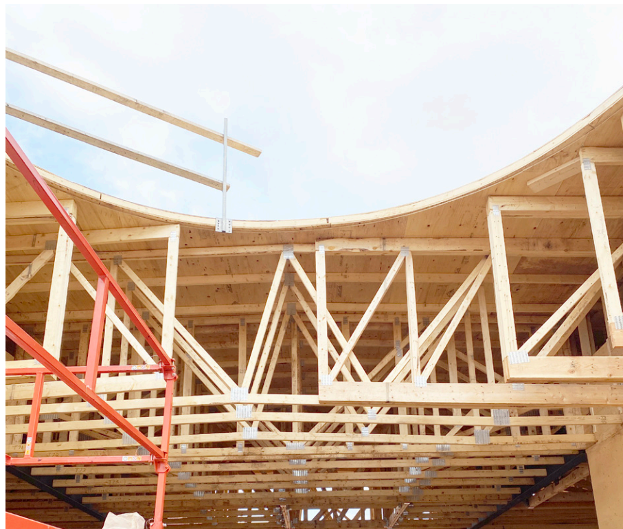
Roof structure in locally harvested pre-fabricated wood trusses
