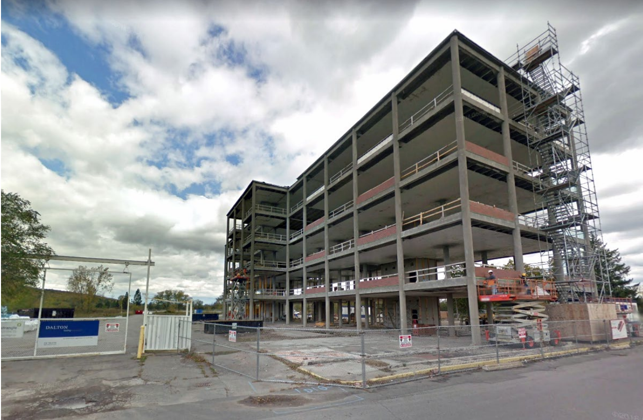
Photos of site with building under construction
