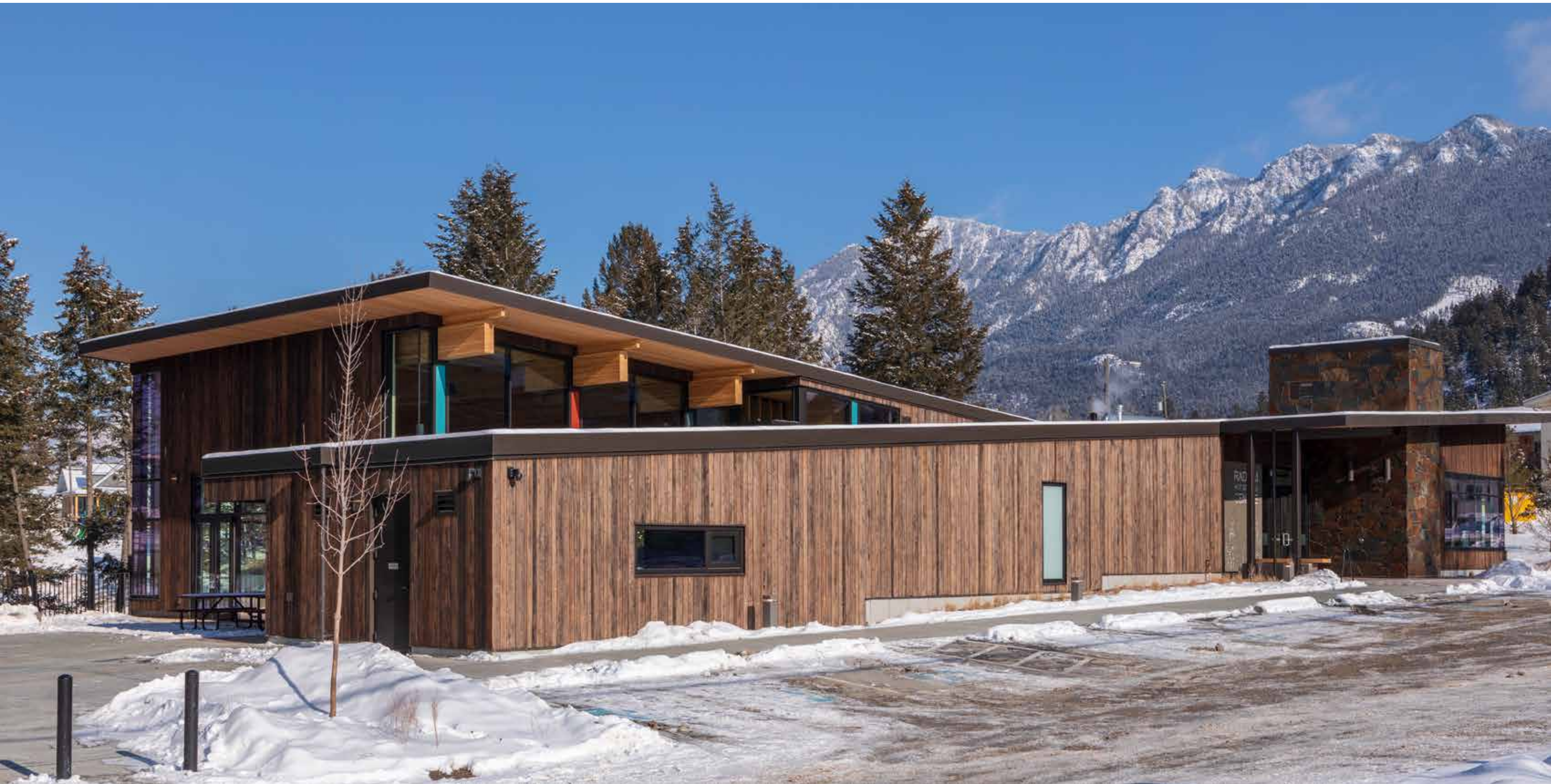
The sloped form follows the natural topography of the site, highlighting views to the mountains beyond.
