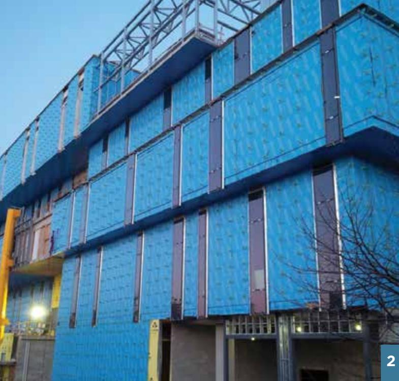
EXTERIOR INSULATION IS AN EFFECTIVE WAY OF ACHIEVING HIGHLY INSULATED WALL ASSEMBLIES, AND CAN SUBSTANTIALLY REDUCE THERMAL BRIDGING AND VAPOUR DIFFUSION [2]. [PHOTO COURTESY RDH]
