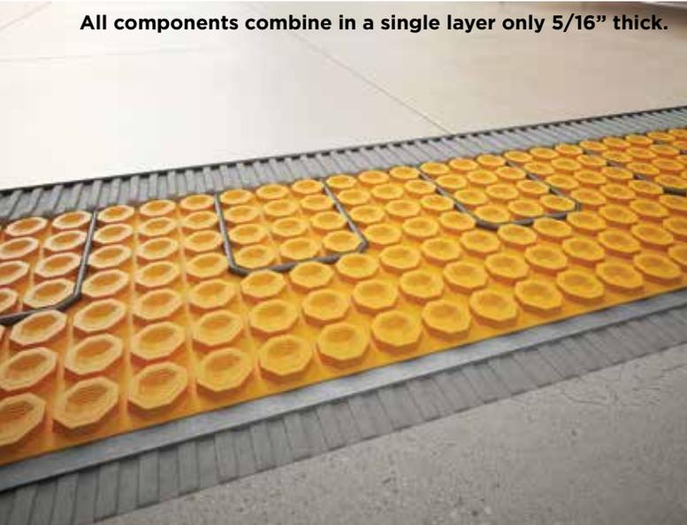
The heating cables snap easily into place.
