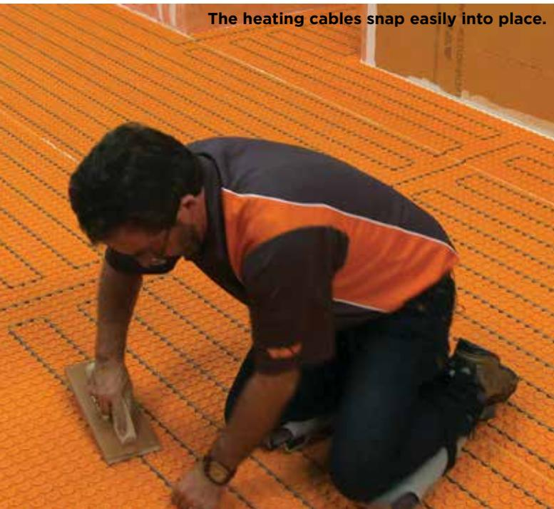
ASTM E2179 testing shows **DITRA-HEAT-DUO** produces an increase in impact insulation class ( $\Delta IIC$ ) of 20 to a concrete slab floor. The dual benefits of reducing impact sound transmission and providing faster warm-up times make this membrane an ideal solution for ceramic and stone tile floor installations in multi-story residential construction.
