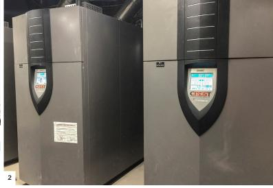
The advanced CREST® introduces a combustion system with a unique burner design with up to 20:1 turndown. The burner fires into an array of 316L stainless steel fire-tubes that transfer the heat to the surrounding water with exceptionally high efficiency.
